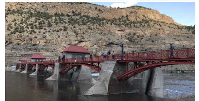
Bridge across a Colorado River reservoir, part of the Upper Colorado River flow enhancement project by Colorado Water Trust.
